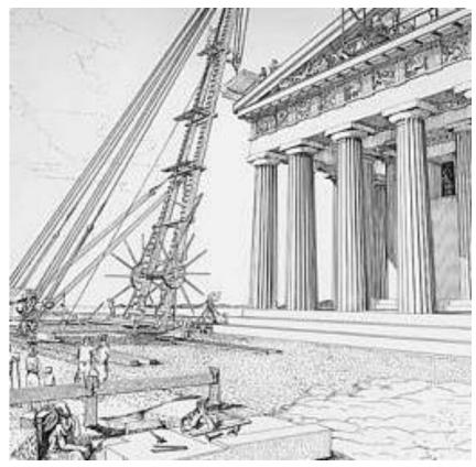
The pulley block and crane made construction of buildings a lot more efficient. This allowed for workers to lift heavier materials. The pulley block and crane were both invented around 515 B.C.
